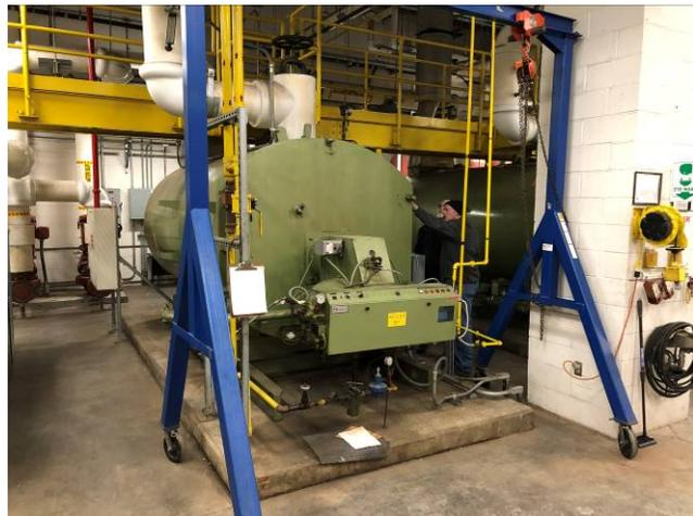
The boilers heat a propylene glycol/water mix that heats the spaces through terminal equipment. Domestic hot water is generated by this same glycol/water mix piped into vertical tank/heat exchangers located in various locations in the building.
