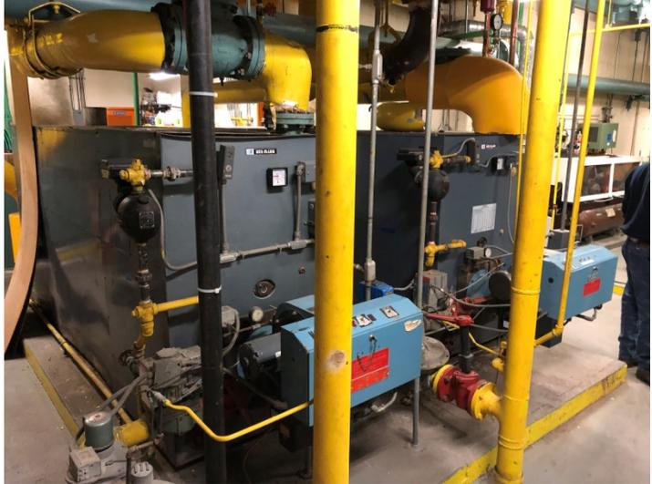
always available when outside air temperature falls below 40°F. The boilers are manually switched from lead to lag. The hot water supply set point for each boiler is linearly scaled as a function of outside air temperature (OAT) as follows: 180°F HWS @ 0°F OAT and 120°F HWS @ 60°F OAT.
